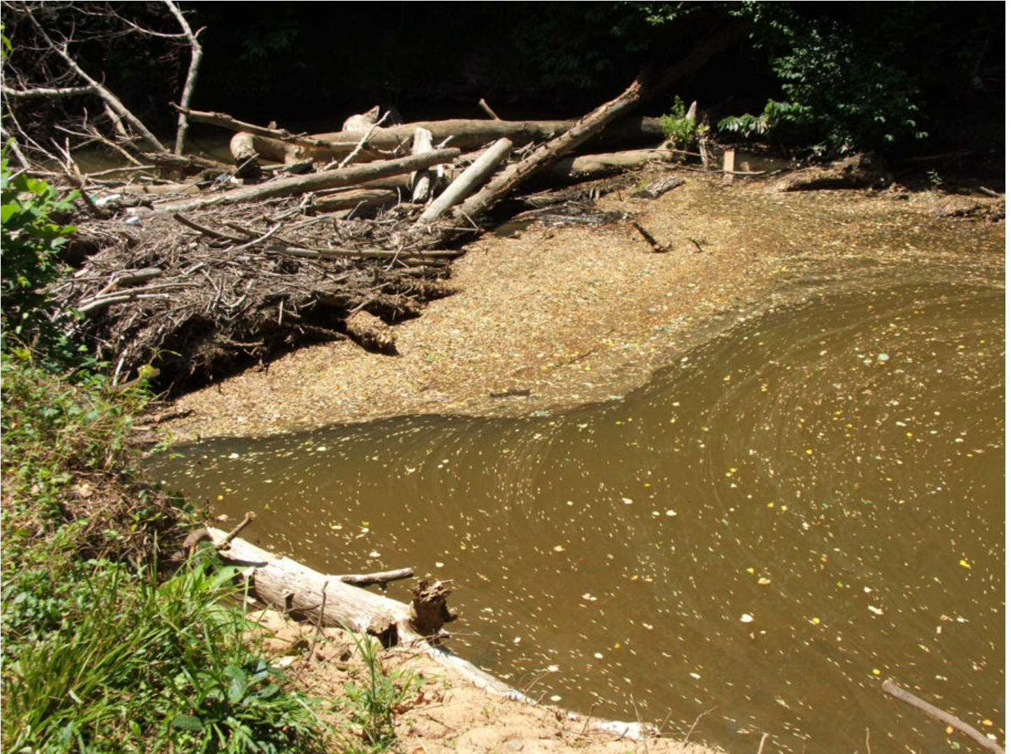
(one of the pictures of the Aquia Harbour Dam)
